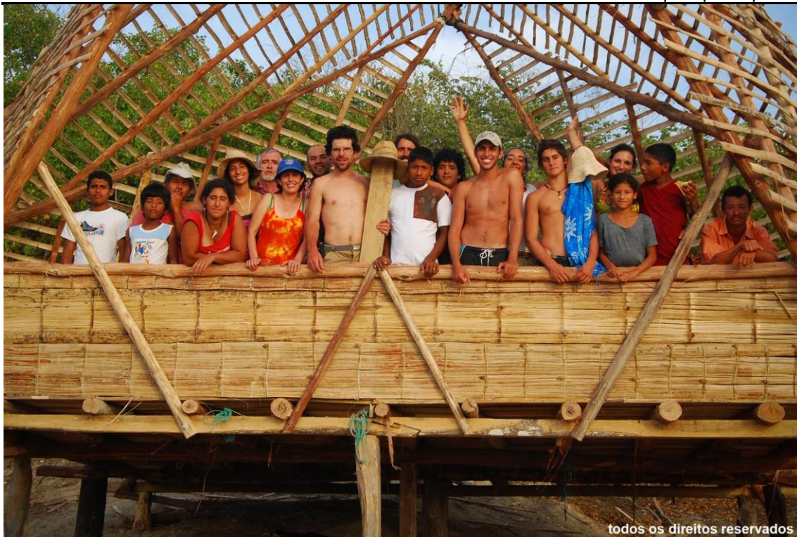
Figure 5 – With the volunteers, during the construction of the Escual Nueva Esperanza
