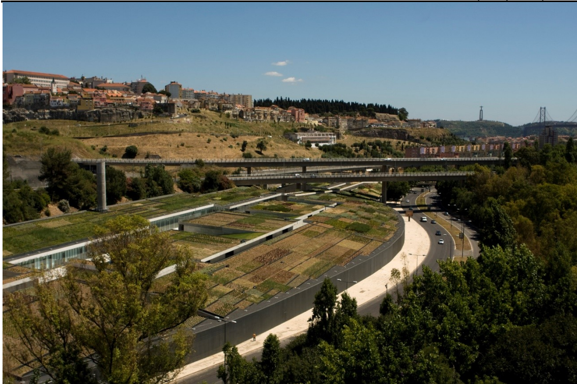
Figure 7 – Alcantara WWTP (Source: PROAP).
