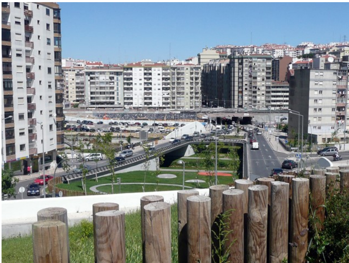
Figure 8 - View of the new roundabout (view from the west). Source: photograph by the author.
