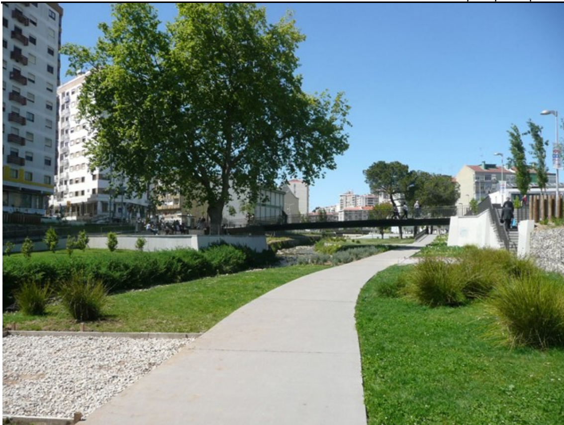
Figure 10 - “Ribeira das Jardas” after the intervention (Linear Park of Ribeira das Jardas). Source: photograph by the author.
